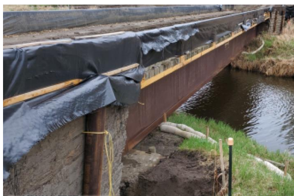
Erosion and sediment control measures in place at Carrot Creek.
