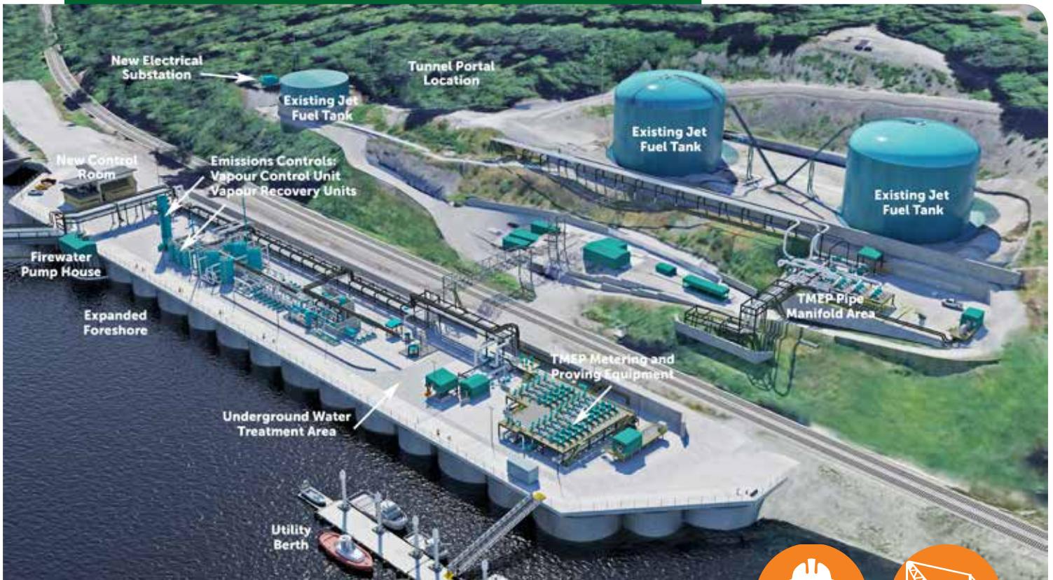
VIEW OF WESTRIDGE MARINE TERMINAL AFTER EXPANSION
