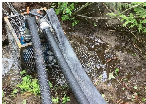
BC 67A watercourse diversion pump and hoses.
