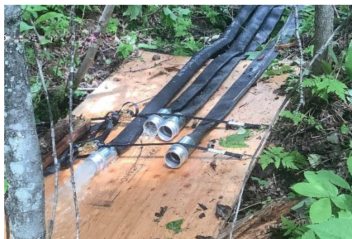
BC 67A watercourse diversion hoses on plywood.
