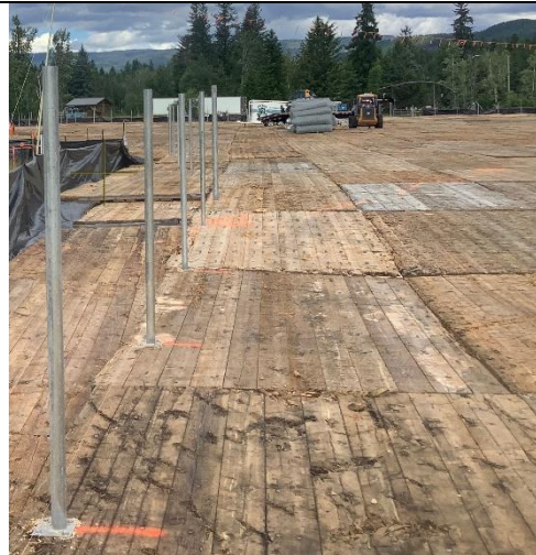
Inspection of wood protective matting at the entrance to the Raft River HDD site.
