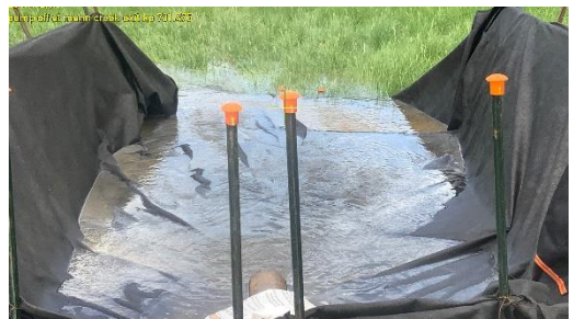
Hydrostatic testing water being discharged at the Mann Creek HDD exit site.
