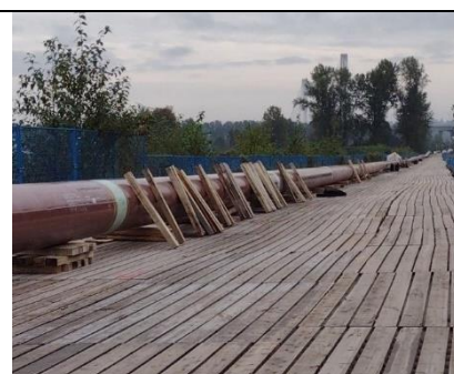
Pipe stored on wooden protective matting on Colony Farm after being welded together. This pipe will be used for the Fraser River HDD.
