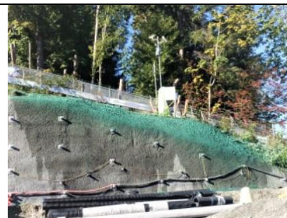
Hydroseed to be covered by poly sheeting at WMT prior to forecasted heavy rainfall.
