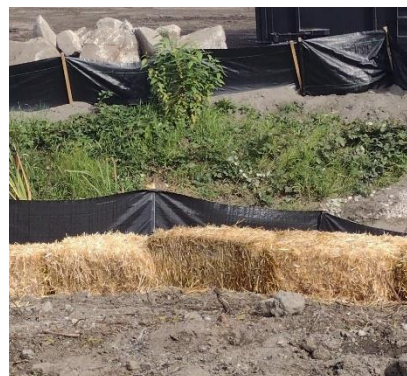
Straw bales and silt fencing functioning as intended at CWP 87.
