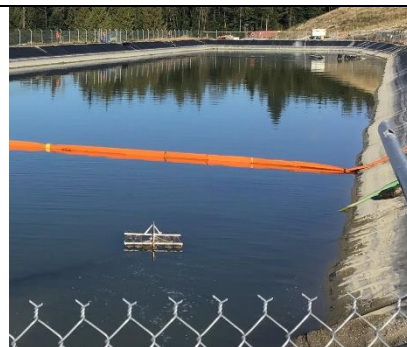
Emptying water from the Intermediate Storm Water Retention Pond (ISWRA) in preparation for heavy rainfall.
