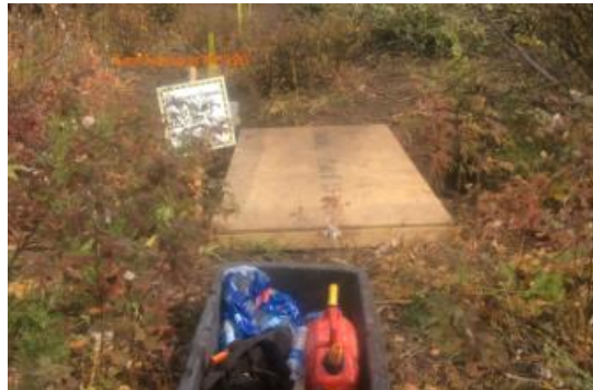
Secondary containment in use near KP 326 in Jasper National Park.
