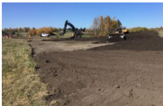
Topsoil replacement KP 41.8.
