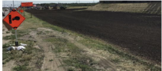
Topsoil restored and ready for seed KP43.
