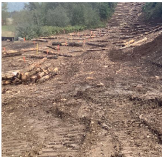
Topsoil and coarse woody debris placed for Oregon Forestsnail habitat near KP 1054.
