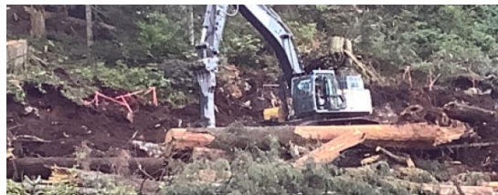
Soil stripping, grading and rock hammer activities monitored near KP 1002.
