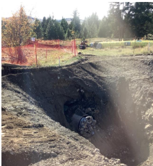
Trenchless construction methods observed at KP 825.
